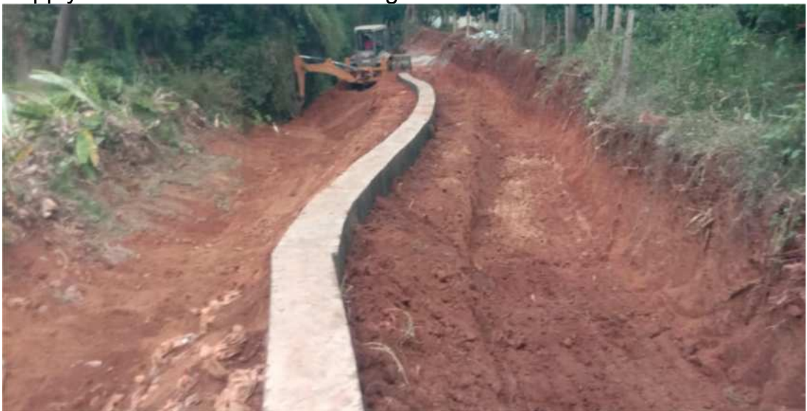
Permanent restoration of Right Side bund at L.S. 50 m to 70 m of Kallikulam Supply Channel in Courtallam Village of Tenkasi Taluk in Tenkasi District
